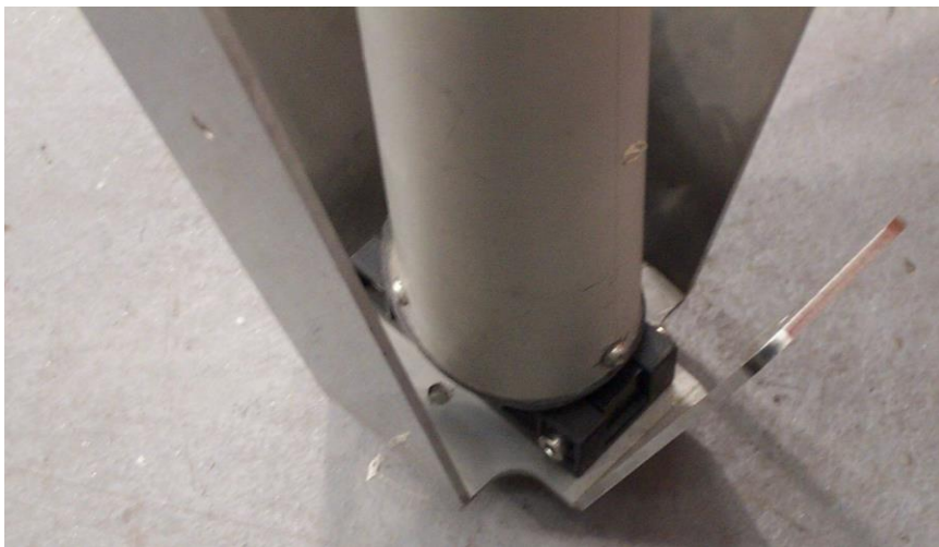
Picture 3.4 The Mast Foot Correctly Located
